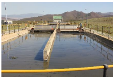
Pasveer Oxidation Ditch
