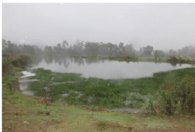
Primary Aerobic Pond No.1
