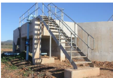
Raised Inlet structure
