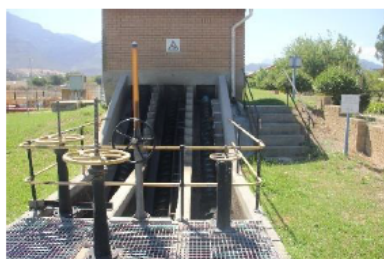
Archimedes screw pumps
