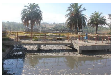
Reactor: Anaerobic zone
