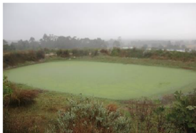
Anaerobic Pond No.1
