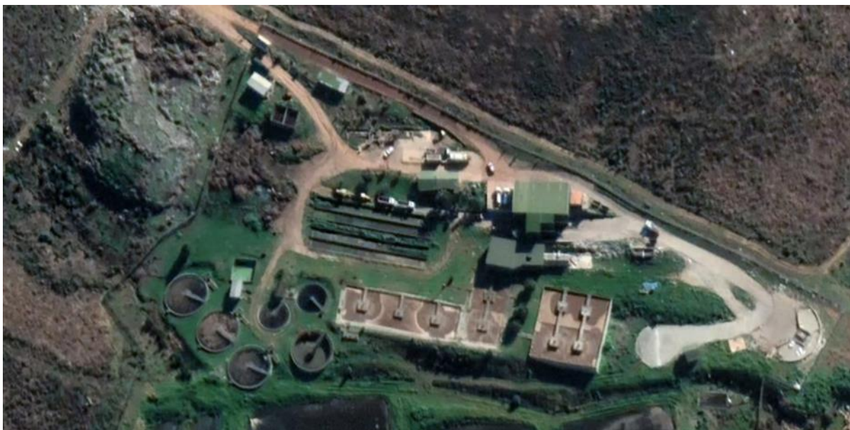
Figure 8 Grabouw Solid Waste Transfer Station
