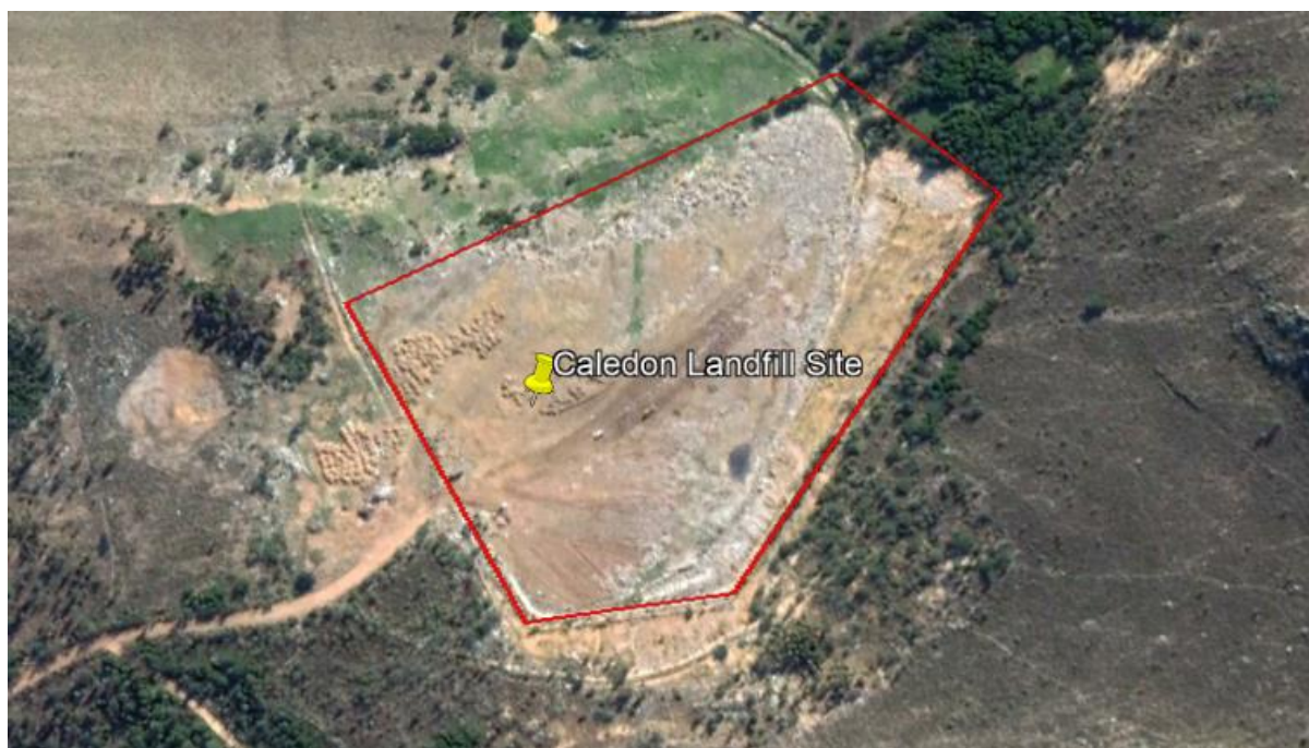
Figure 10: Caledon Landfill site
