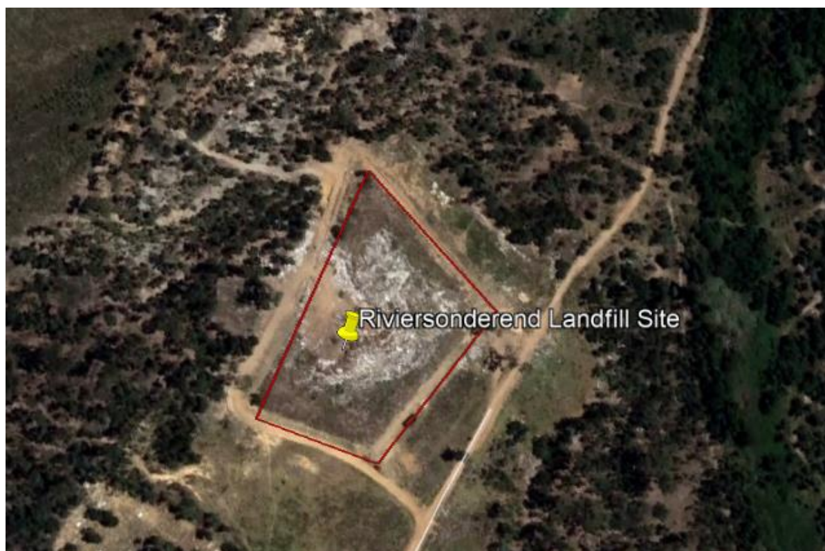
Figure 13: Riviersonderend (RSE) Landfill site
