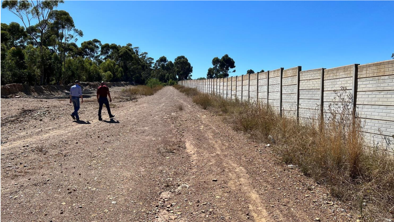
Figure 2: Access road to be upgraded
