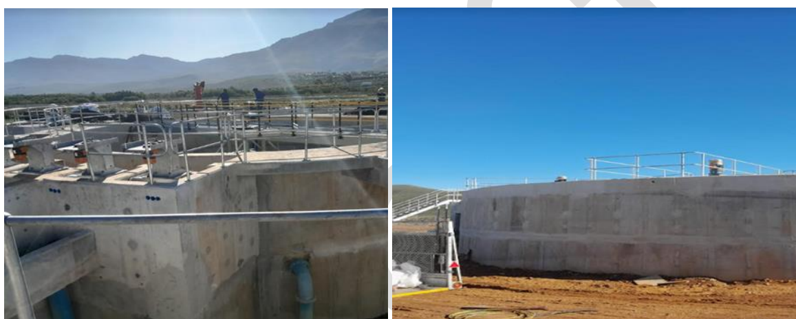
The Newly constructed Greyton Wastewater treatment.
